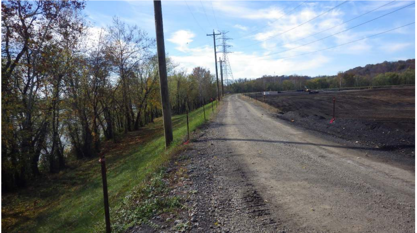
Photograph 17 – Eastern embankment with boiler slag closure area on the right.
