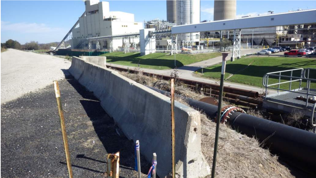
Photograph 1 – LVWTS piping entering southeast corner of the SFAP embankment.
