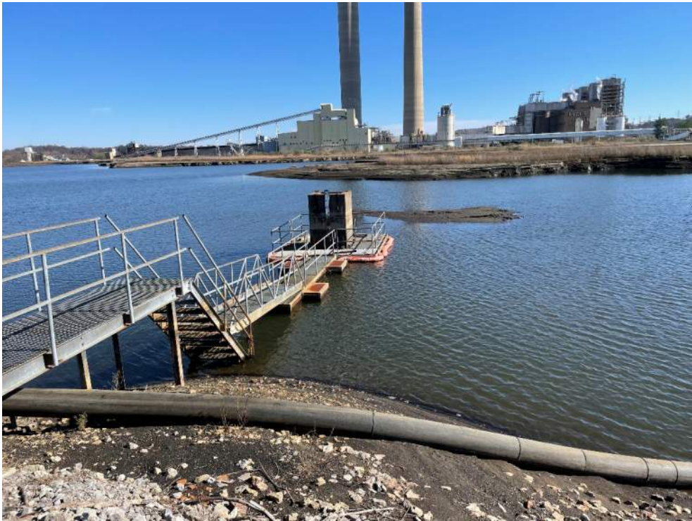
Photograph 15 – Outlet structure in southwestern corner of SFAP.
