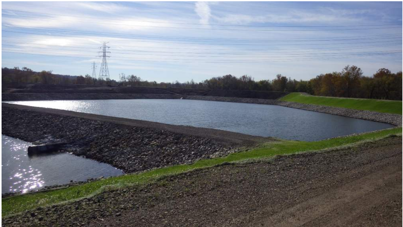
Photograph 4 – New vegetation along western and southern side of LVWTS, secondary basin.
