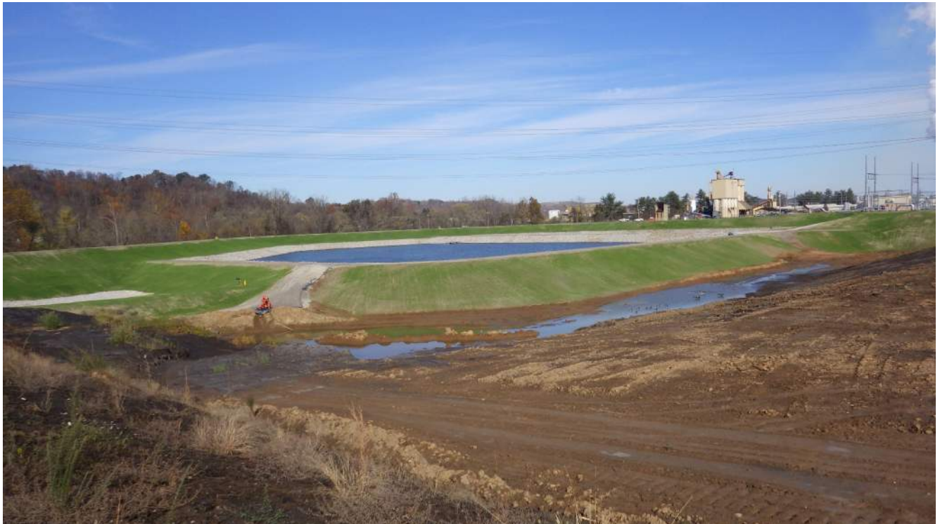
Photograph 10 – BSP water management and pumping adjacent to LVWTS.
