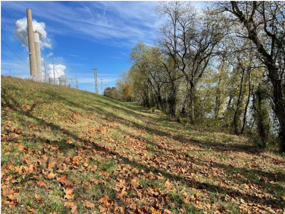
Photograph 14 – Downstream eastern embankment of the BSP.
