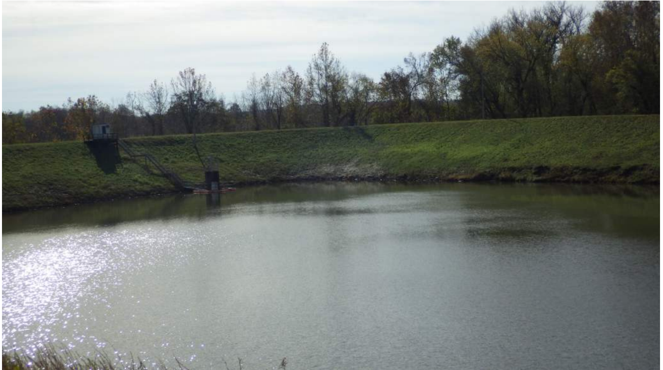
Photograph 11 – Outlet structure from Clearwater Pond to the Ohio River.
