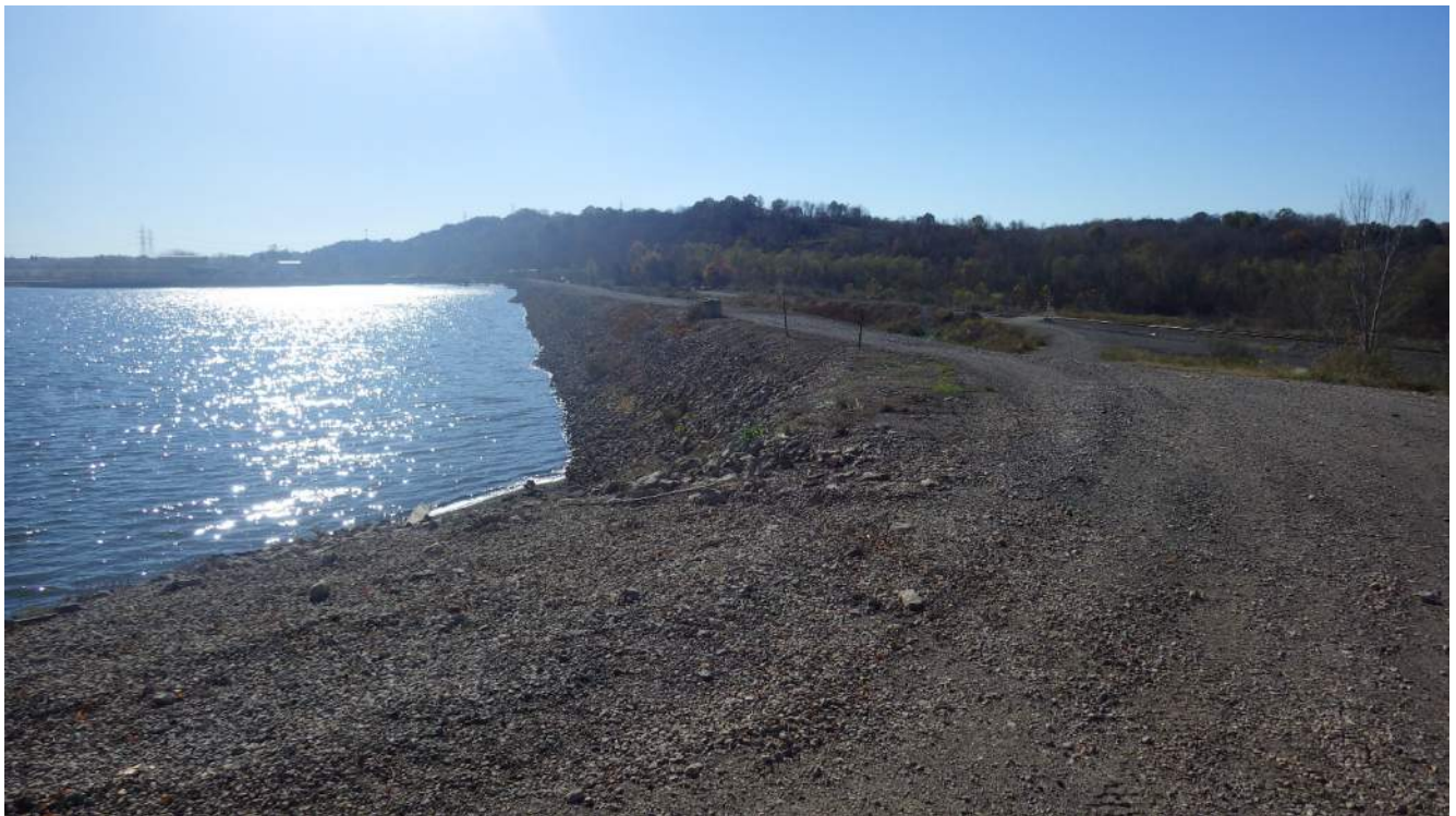
Photograph 12 – Western embankment showing upstream riprap protection.
