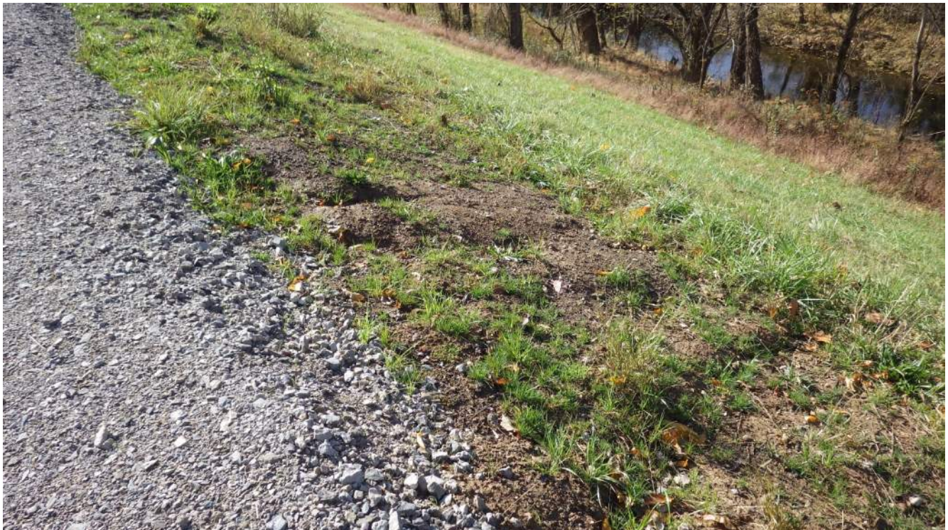
Photograph 6 – Bare spot located on slope between BSP and Kyger Creek.
