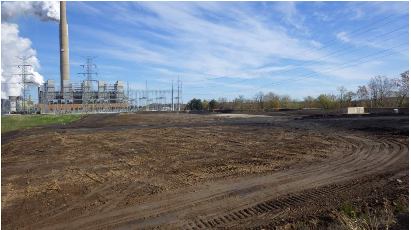
Photograph 12 – Boiler slag pond closure area east of LVWTS.
