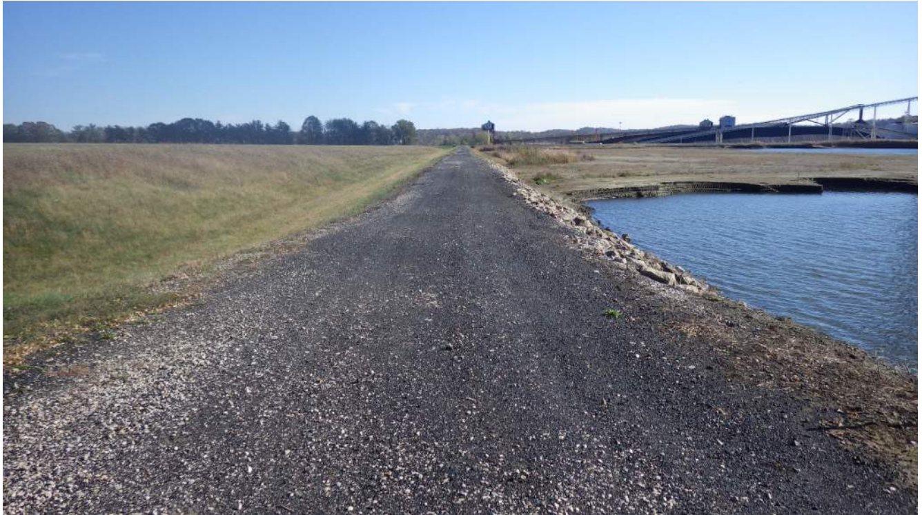
Photograph 11 – Northern dike showing upstream riprap protection.
