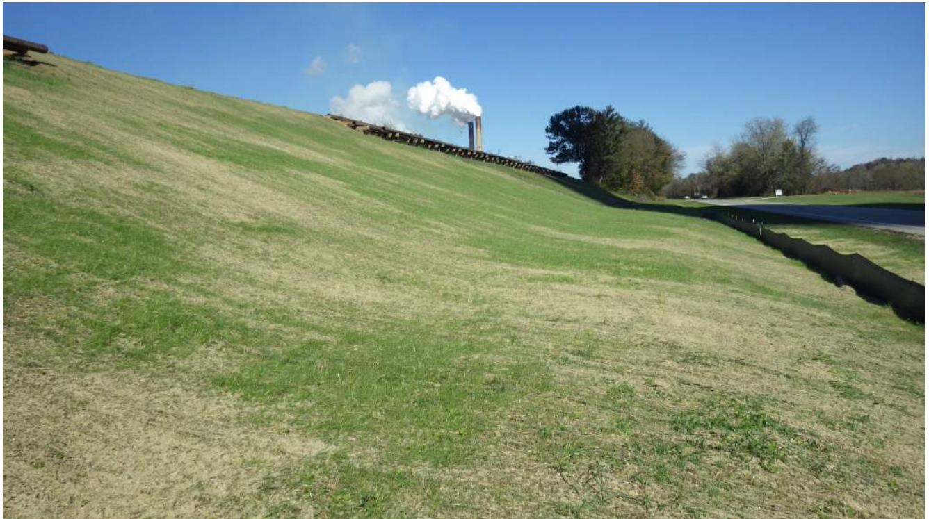
Photograph 8 – New vegetation at possible LVWTS piping crossing on downstream side eastern embankment.
