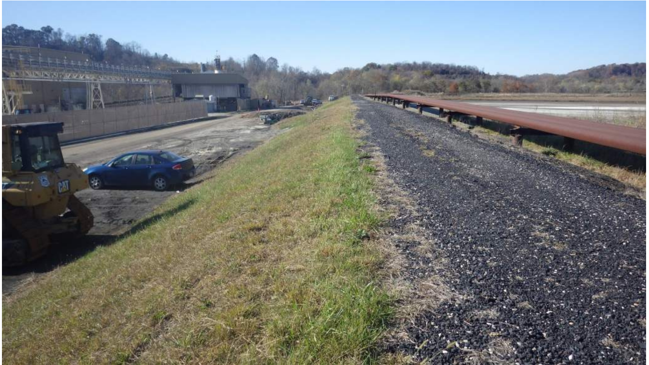
Photograph 17 – Downstream side of southern embankment. Construction near area toe was excavated.
