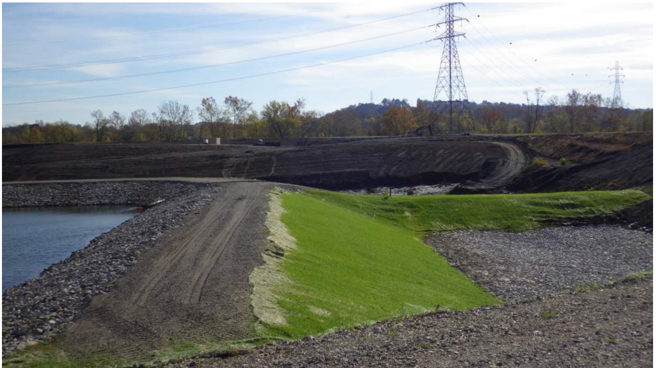
Photograph 8 – New vegetation on southern LVWTS dike, secondary basin.
