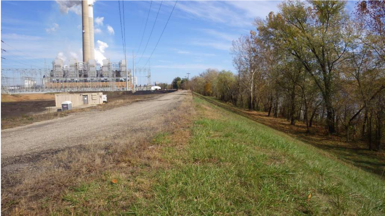
Photograph 13 – Downstream eastern embankment of BSP.
