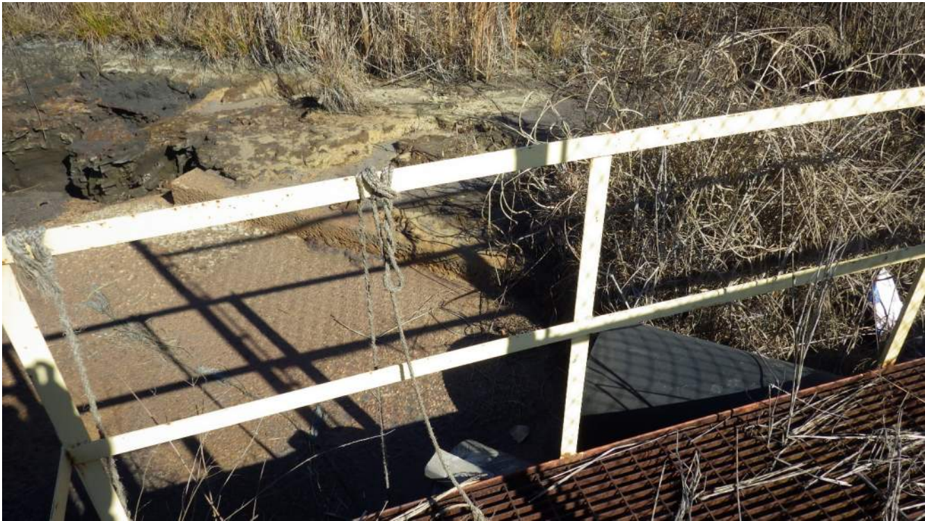
Photograph 2 – Southeast inlet into SFAP.
